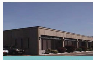
CTDOT completed demolition of 88 State Street for commuter parking.
